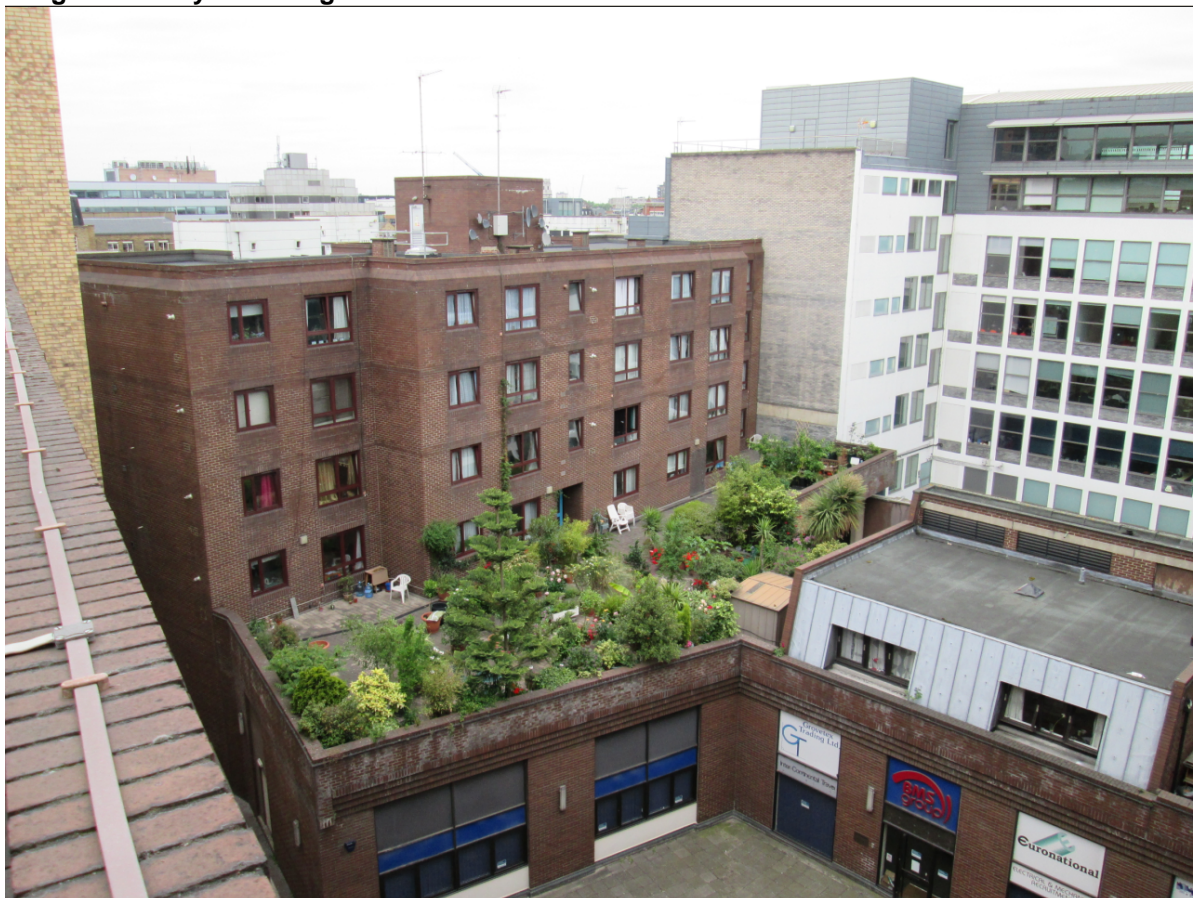
Image 4: Rear courtyard facing elevation of 10 Epworth Street with first floor terrace garden.
